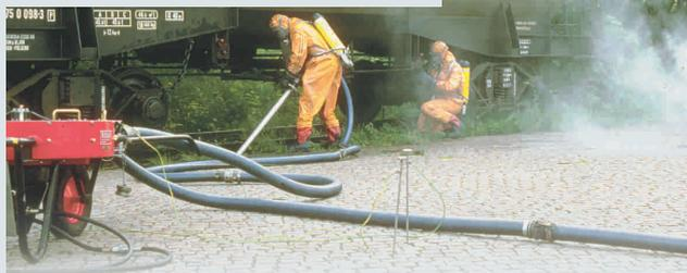
The standard inner lining of the pump hose is made of nitril for long term pumping of oil but the material can also handle short term operations of a number of aggressive chemicals. The risk for sparks is very small as the power pack can be placed outside the hazardous area and the rotating speed of the pump is very low. Also the system can easily be grounded to earth.
